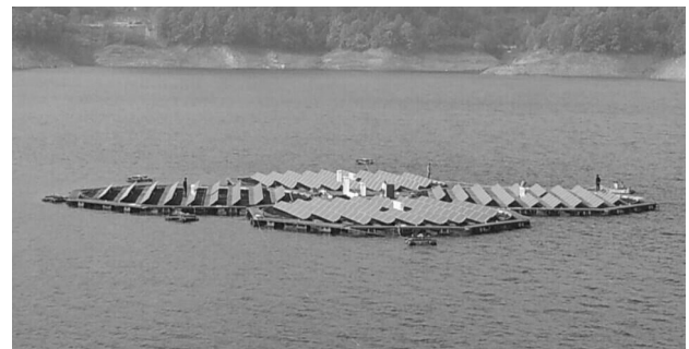
Fig. 15 Tracking-type Floating PV Generation System
