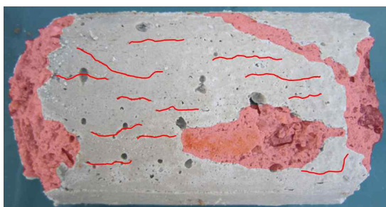
Figure 5. Surface erosion of alkali-activated hwangtoho concrete owing to chemical attack ( t_c=91 days)
