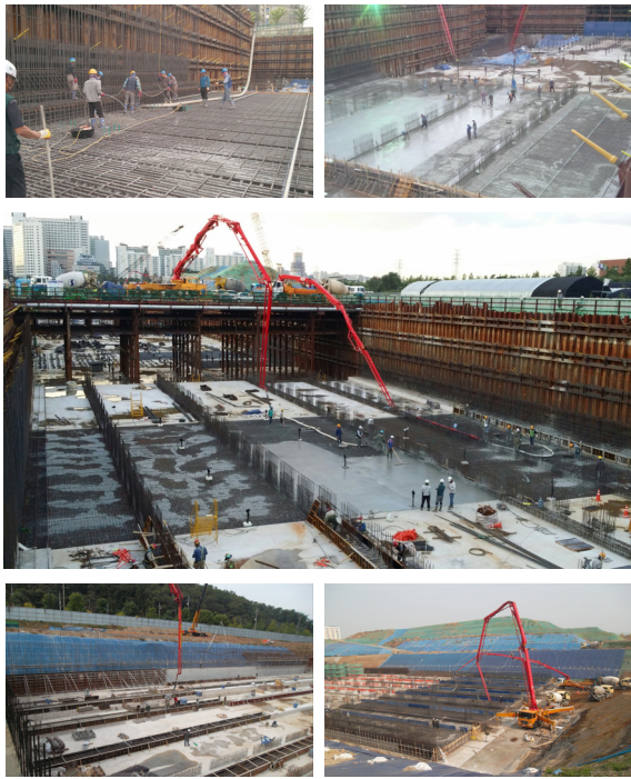
Fig. 16. Field applications of concrete with Premixed Cement
