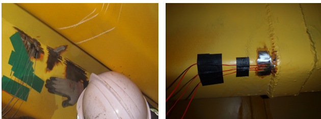
Fig. 10 IIW installation of Strain gauge (2st test)
