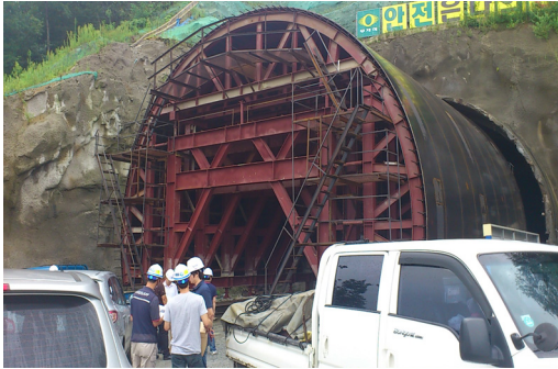
(a) Entrance of tunnel
