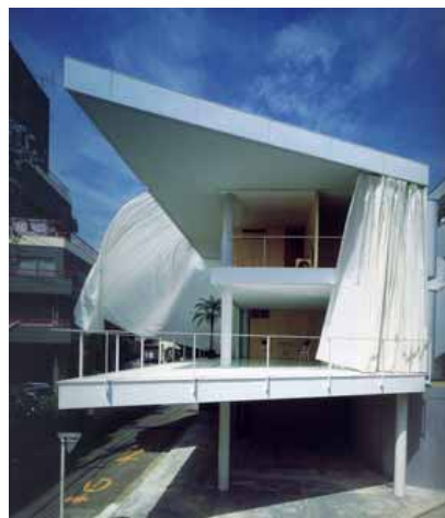
Figure 2. Curtain Wall House, Shigeru Ban - http://www.designboom.com
