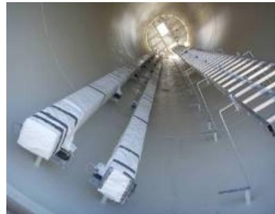
Fig. 6 Bus duct installation on tower section
