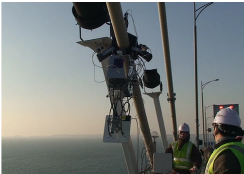
Fig. 14 Field test for performance of cable climbing robot
