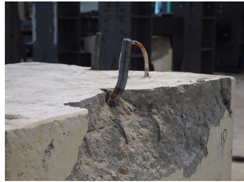
Fig. 16. Typical concrete fracture of stirrup reinforced anchor
