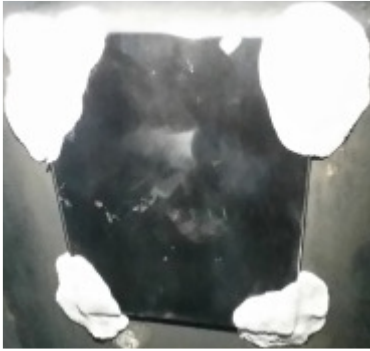
Fig. 3. Iron plate sticking on the heating surface of the combustion chamber
