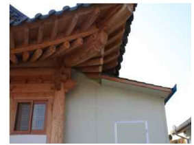
Figure 22. The rear extension
