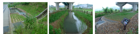
① Small Constructed Wetland ② Free Water Surface Wetland ③ Horizontal Sub-Surface Flow Wetland
