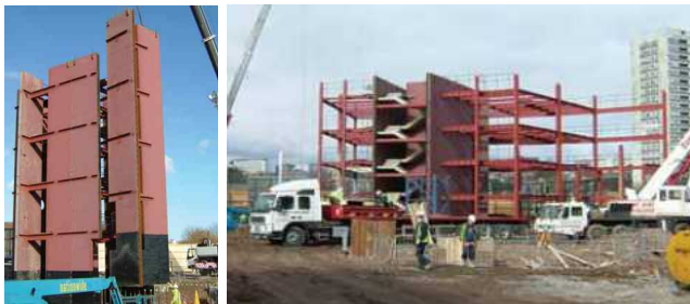
Figure 2. Birmingham 1 tower (Bi-steel)
