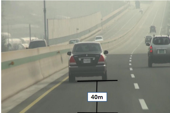
Fig. 2 Investigation of Vehicles' Lateral Wheel Paths
