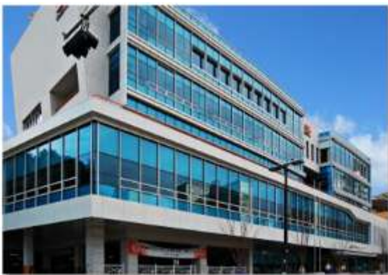
Fig. 13. View before the installation of solar control system
