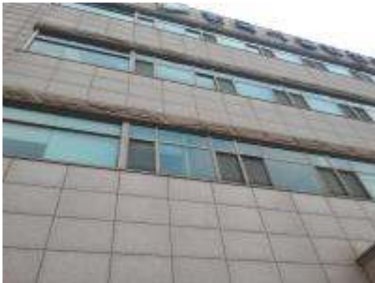
Fig. 3. View of external wall of building
