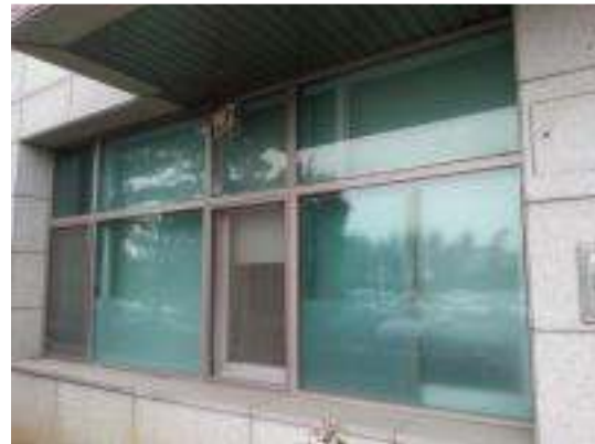
Fig. 4. View of the window installation
