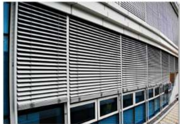
Fig. 14. View after the installation of solar control system
