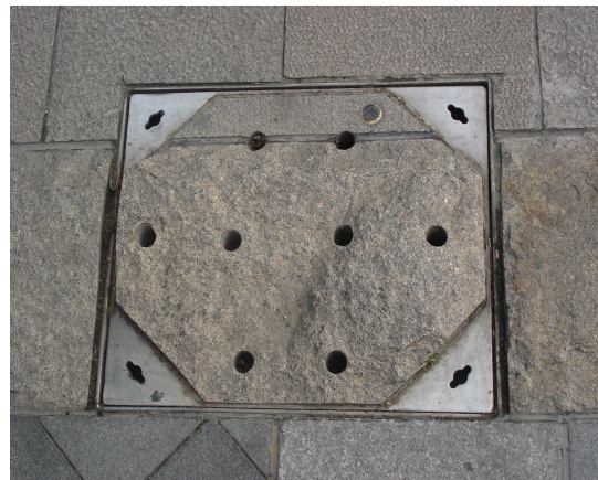
Fig. 3. The Well Covers Integrated With the Pavement.
