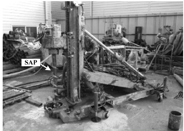
(b) Installation of 1 st SAP
