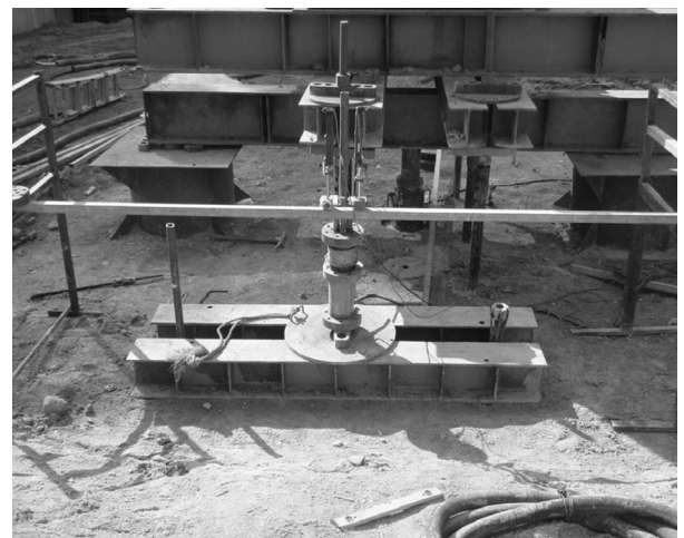
Fig. 7. Field pullout test setup
