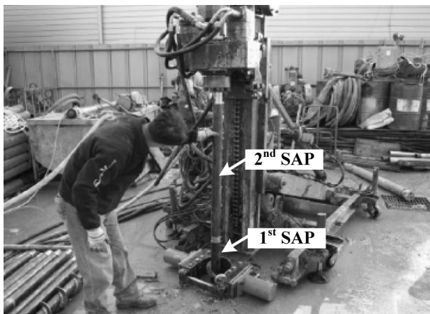
(c) Installation of 1 st and 2 nd SAP
