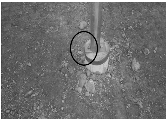
Fig. 8. Location of baseplate in footing.
