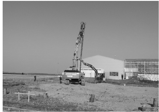
Fig. 7. Wood pile driving.
