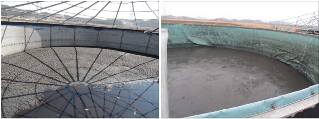
Fig. 1. Surface of sediment layer in liquid fertilizer storage tank.
