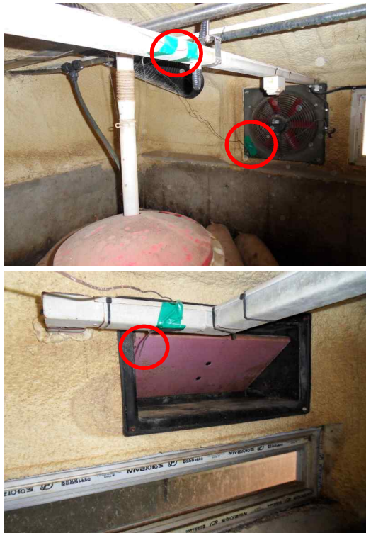
Fig. 3. The sensors for temperature in pen.
