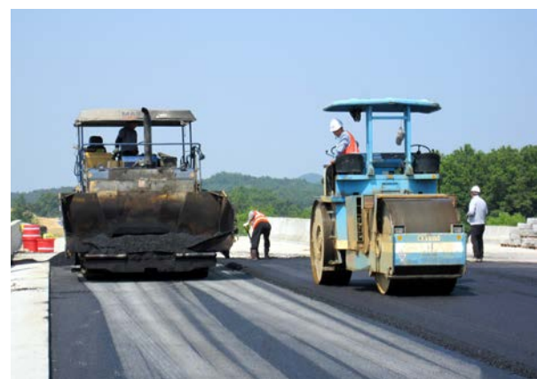
Fig. 2 Pick up of Tack Coat Materials by Construction Truck
