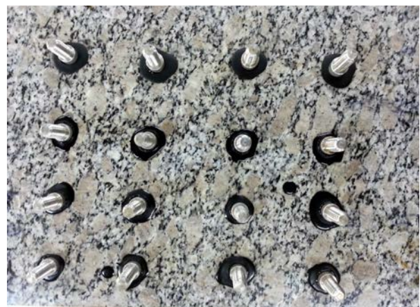
Fig. 9 Preparation of Pull-out Stub by PATTI
