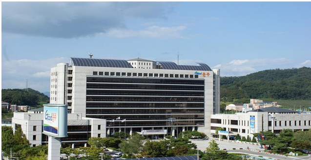
Fig 1 Photovoltaic system of C city hall
