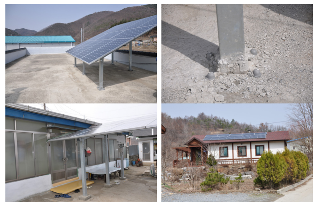
Fig. 2. Condition of the surveyed facilities
