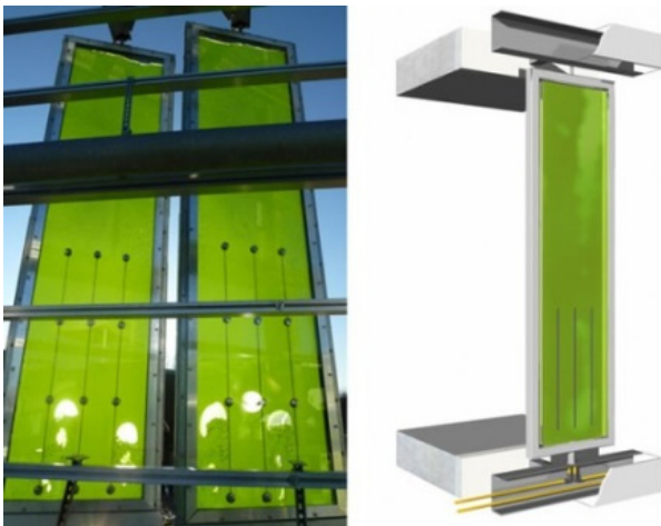
Fig. 4 Case model for algae facade in Hamburg, Germany (Source: International Building Exhibition)
