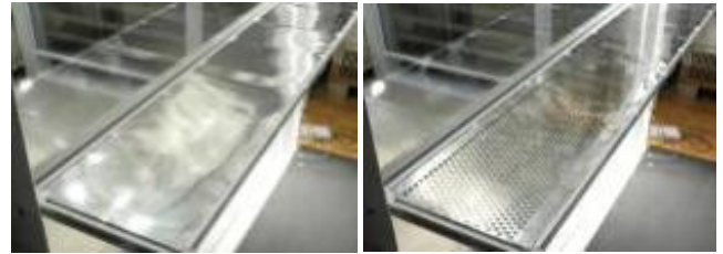
① Light Shelf which has not been applied ② Light Shelf which has been applied Fig. 4. Light Shelf applying punching plate
