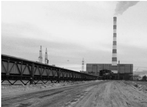
Fig. 1. Coal deliveries for Berezovskaya GRES using the overland belt conveyor CML-4500 (stack height of 370 m)
