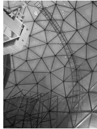
Figure 2. Installed ladder inside radome.
