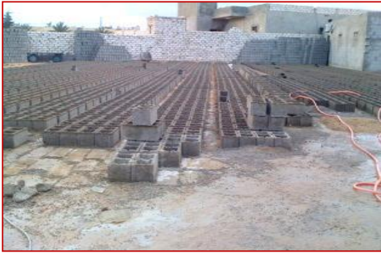
FIGURE IV Manufacturing of cement blocks, 02.2013. Source: author.
