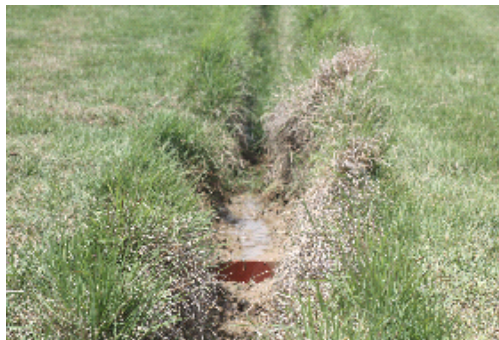
[Fig. 3] Runoff water collector installation.
