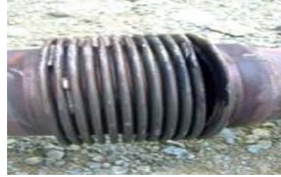
Figure 2: Early failure due to fracture
