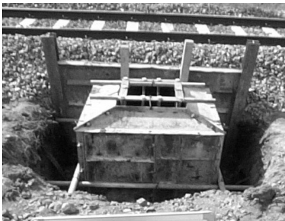
Fig. 2. Interference of railroad track due to excavation for pole foundation
