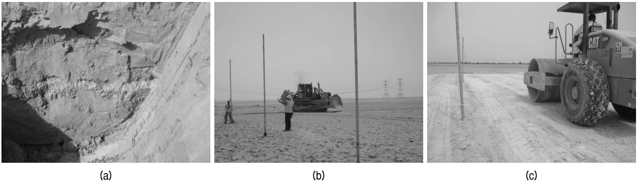
Fig. 6. Test Embankment in Sabkha area with ground-water level of GL-0.5~-1 m
