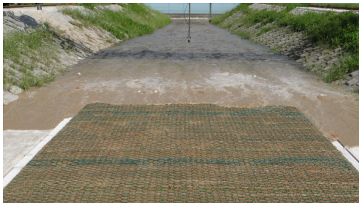
[Fig. 5] Installation of vegetation mats
