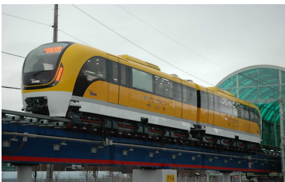
Fig. 1 Maglev vehicle running over the elevated guideway
