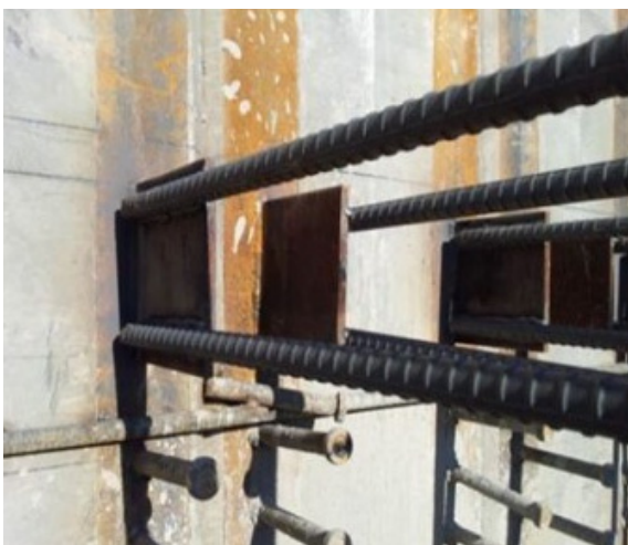
Fig. 4 Example of moment plate connection
