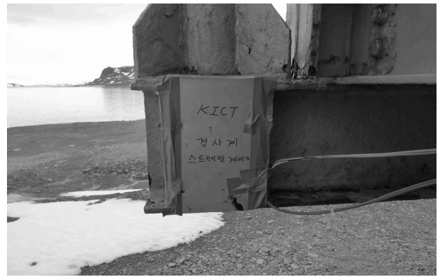
Fig. 7. Monitoring sensor system installed in marine biology laboratory
