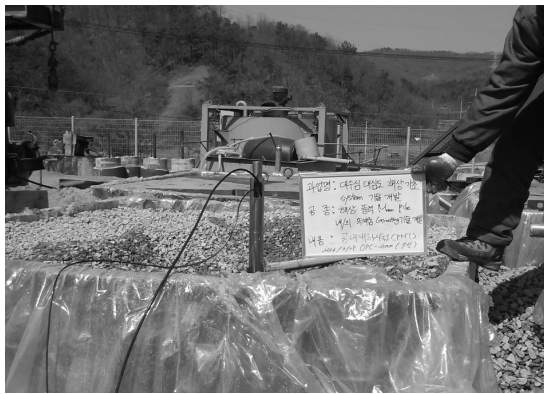
Fig. 6. Panoramic view of pressuremeter test
