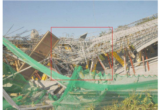
(a) Right view of girder
