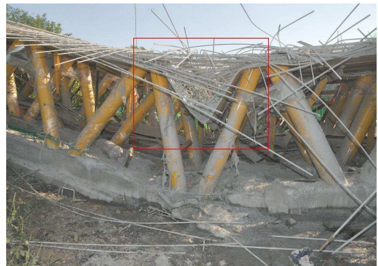
(b) Left view of girder
