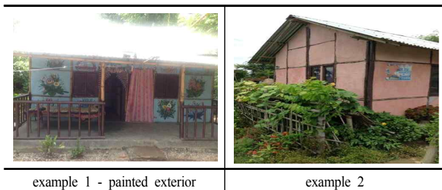
Fig. 4. Example of houses provided by Habitat for Humanity, Nepal
