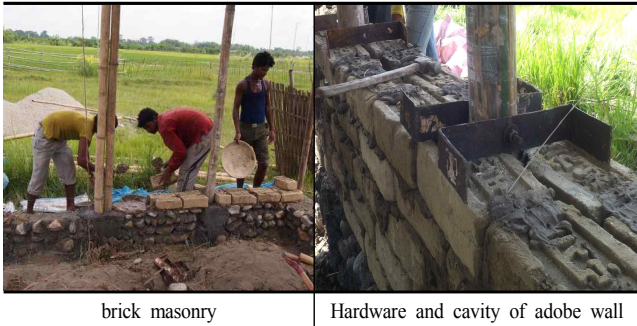
Fig. 10. Construction of adobe Brick House
