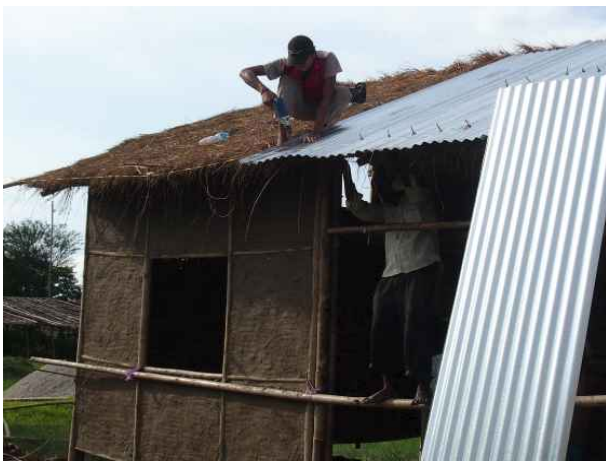
Fig. 6. Installation of straw mat under CGI Sheet
