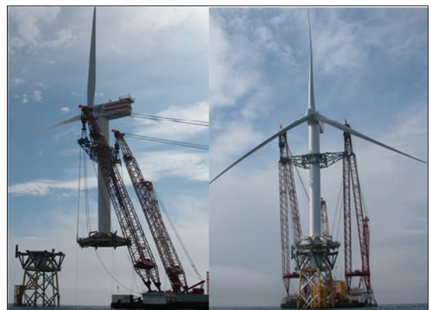
Fig. 2 Installation of offshore wind turbine using floating crane ( http://www.scaldis-smc.com/beatricewindfarm.html )
