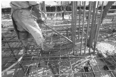
Figure 17. Concrete pouring to slab-column connection
