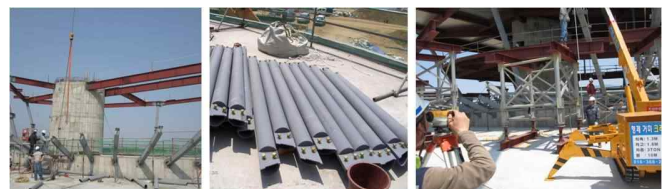
Figure 14. Field assembly and 3D coordinates check
