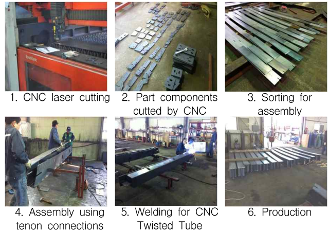
Figure 11. Components fabricating process for steel beam structure
