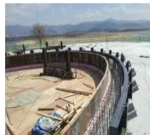
Figure 12. Template plate construction for basic point control
