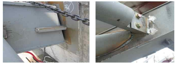
Figure 7. Connection details of the steel beam structure
