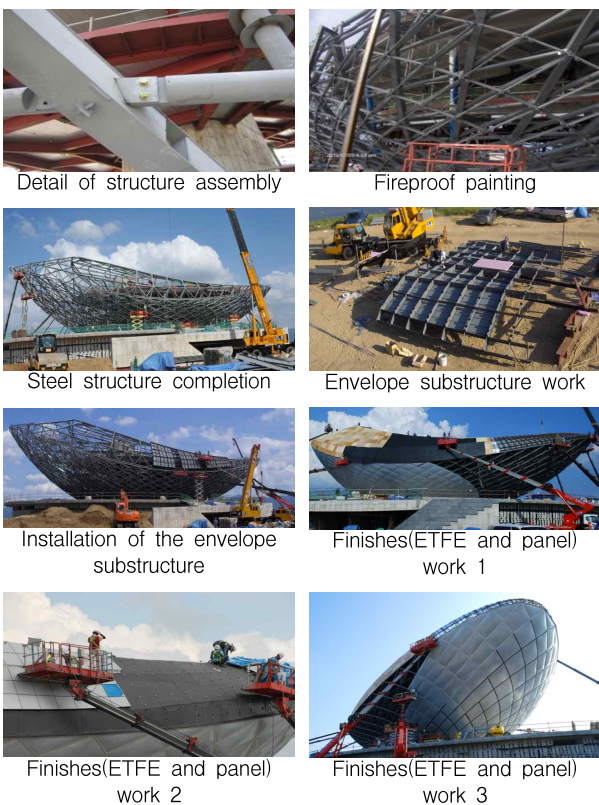
Figure 15. Manufacturing and construction process of The ARC
