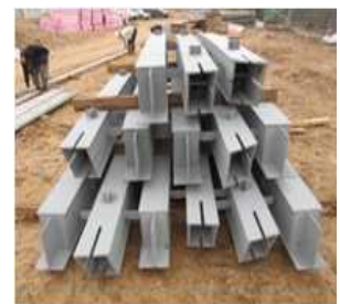
Figure 13. Field load of the steel beam structure
