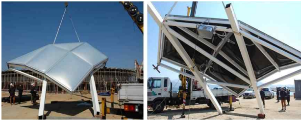
Figure 9. Field mock-up of structure and finishes(ETFE)
