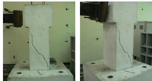
〈Fig. 8〉 Crack patterns (Ref. Experimental reinforcement)
