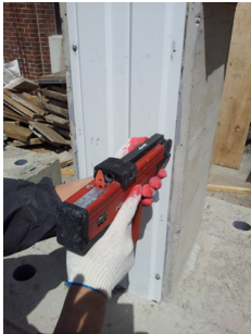
(3) Power pin installation
