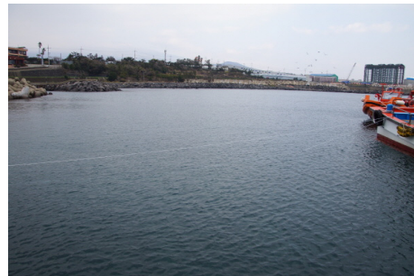
[Fig. 14] Nylon rope test at quayside
