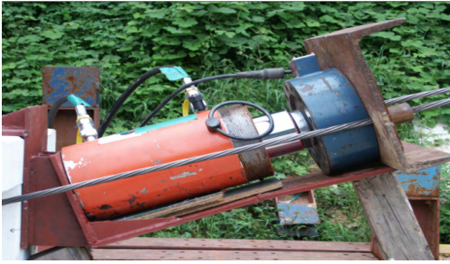
Fig. 8 End anchorage and measurement of prestressing force using a load cell
