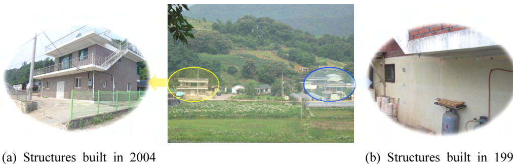
Fig. 2 Sampling place of concrete structures
