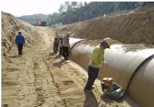
(e) First Layer Backfill
