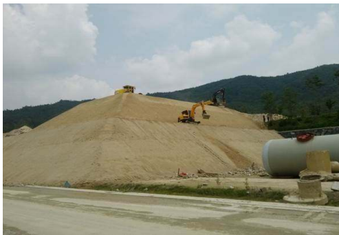
(f) Second Layer Backfill and Completion
