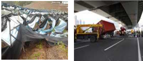
Figure 1. Wind Gust Damages
