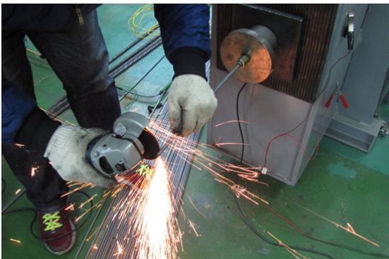
Fig. 10. Section cutting of PS wire after stressing
