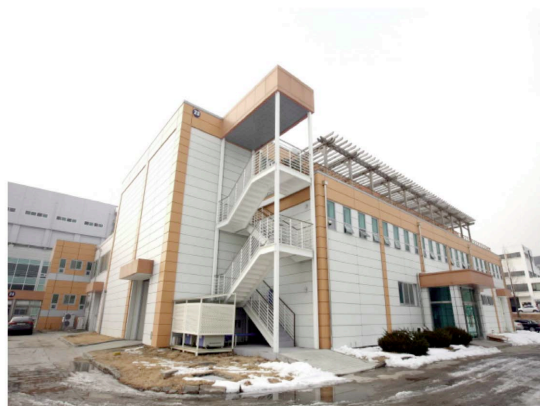
Fig. 7. The PRIDE Experimental Pyroprocessing Facility in Daejeon.
